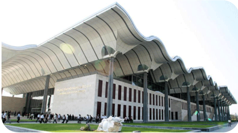
Electrical accessories for National Assembly Building and National Convention Centre
