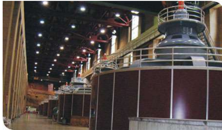
Cables for Thac Ba Hydropower plant
